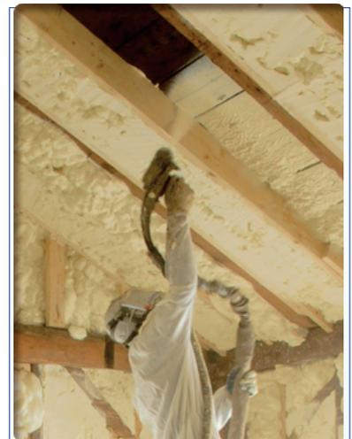
*Spray foam can be installed in both new and existing homes, and even in the most unusual designs. It adheres to wood and steel frames alike and is effective in any climate. When you put spray foam anywhere in your home, the general benefits apply, but there are also additional reasons to use high performance insulation in very specific parts of a home.*
